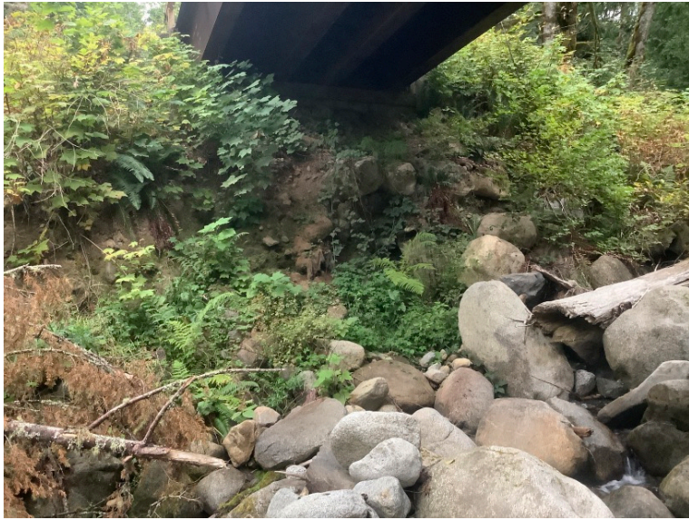
Right Bank Abutment when facing downstream
