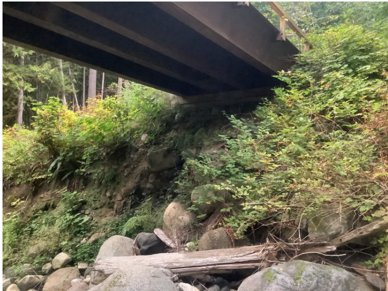
Right Bank Abutment when facing downstream
