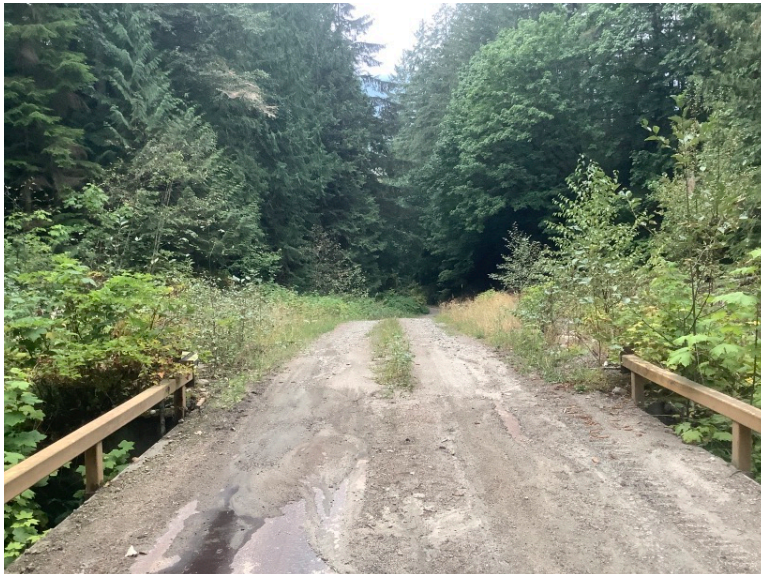
Bridge deck, viewing to left approach
