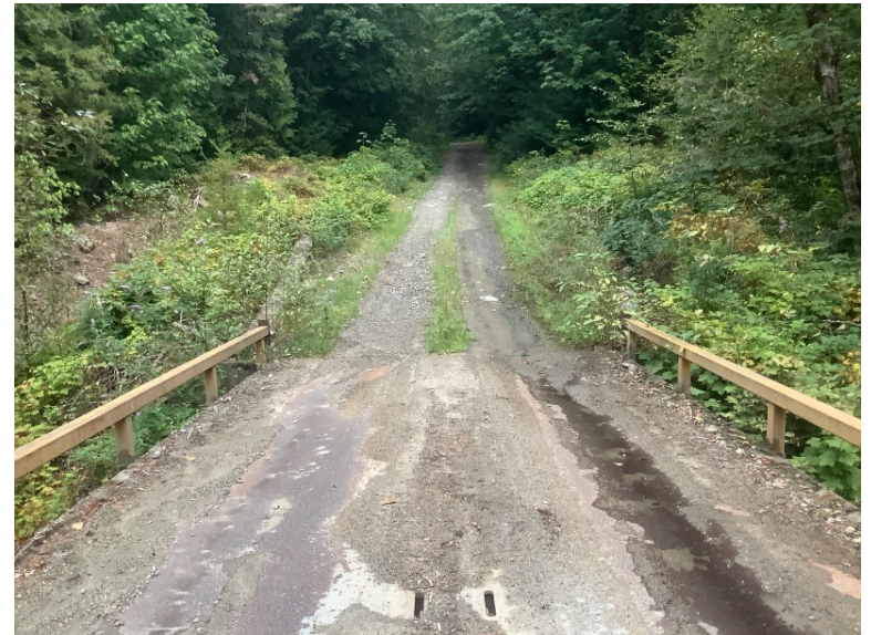
Bridge deck, viewing to right approach
