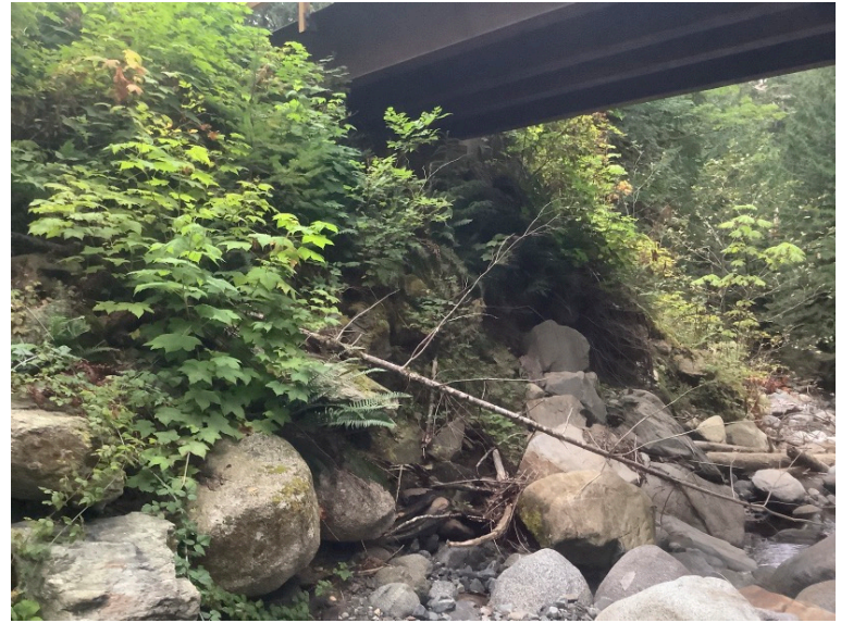
Left Bank Abutment when facing downstream
