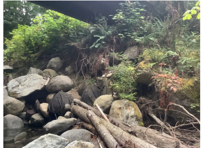
Left Bank Abutment when facing downstream
